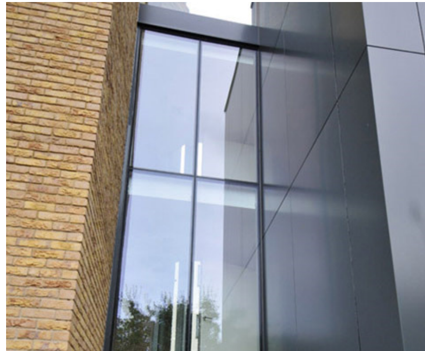
Fig. 19: Image of Curtain Walling
